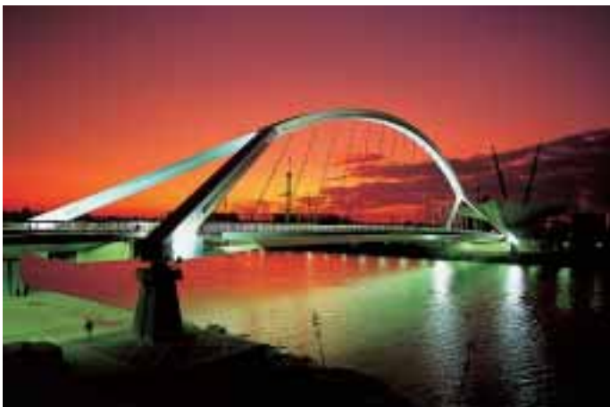
La Barqueta Bridge
